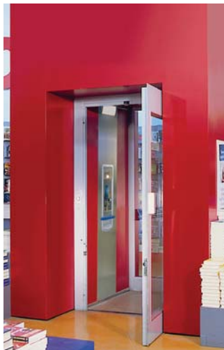
Platform with hinged door opening on right in masoned shaft.
